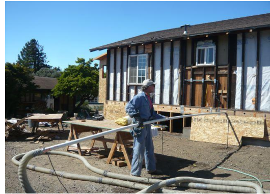
Blowing insulation into the Blue House retrofit
